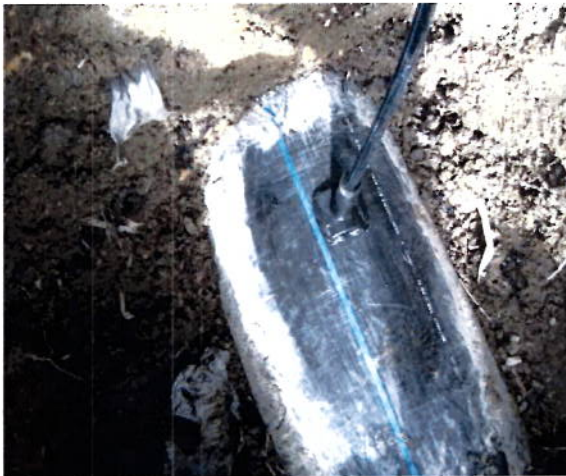
EMPALME TUBERIA PVC A AC
