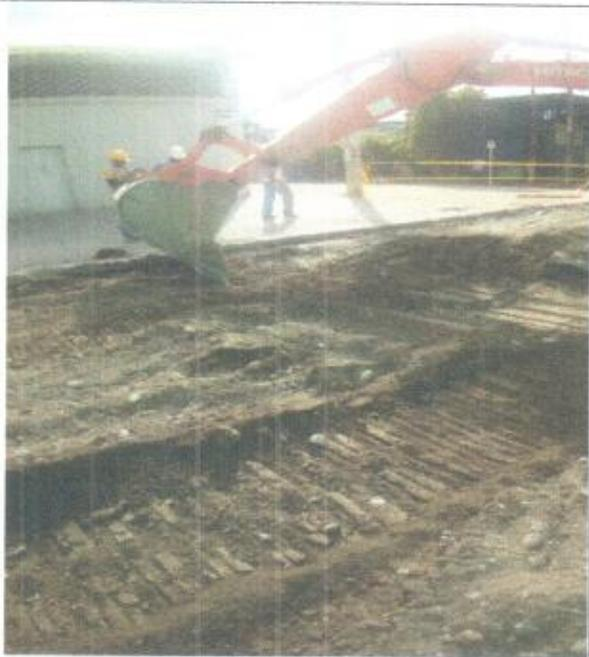
**SE EVIDENCIA DOBLE LOSA DESPUES DE LA
