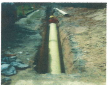
PHOTO 10: Laying of concrete pipe in trench.
