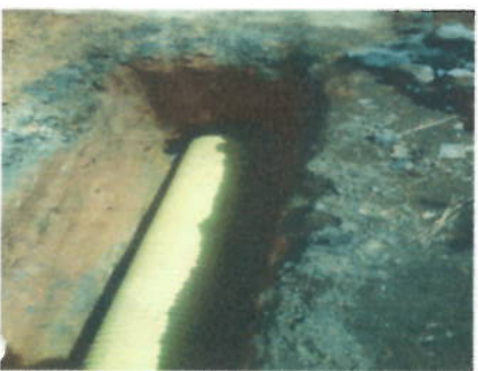
PHOTO 10: Laying of concrete pipe in trench.
