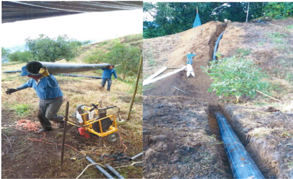
ACARREO TUBERIA AL HOMBRO – TUBERIA INSTALADA
